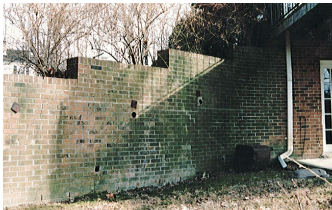
Brick Wall Joins House wall
